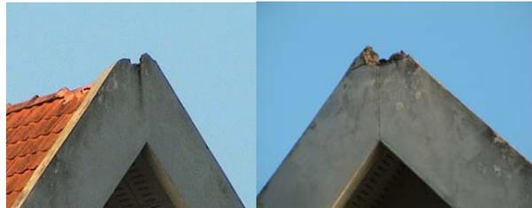
Fig. 3. Close-up photographs of the lightning damaged ridge ends.
