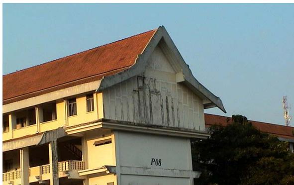
Fig. 1. The UTM electrical engineering building (Block P08) that was struck and damaged by lightning at the southern ridge end.
