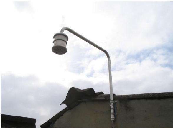
Fig. 4. Electric field mill
