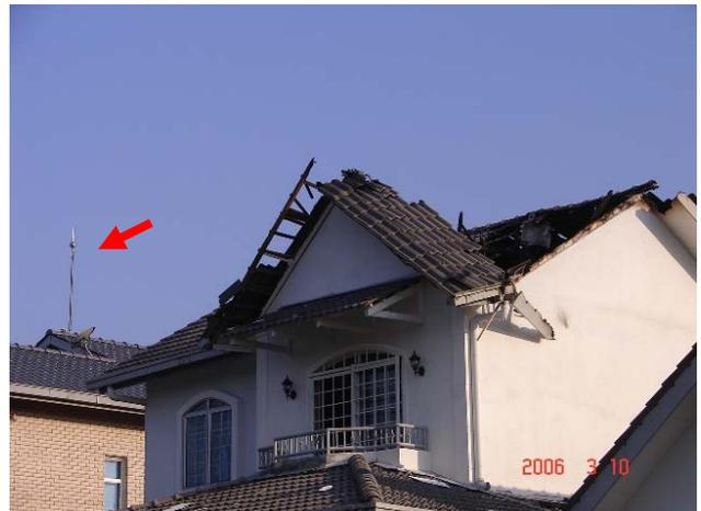
Fig. 2: Close-up view of the ESE air terminal (arrowed) on the adjacent house.
