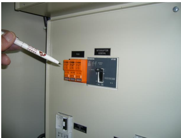
7. DIN-Rail Mounted SPD
